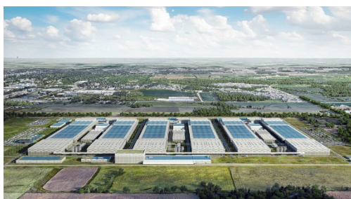
The future PowerCo cell plant in St. Thomas, Ontario
